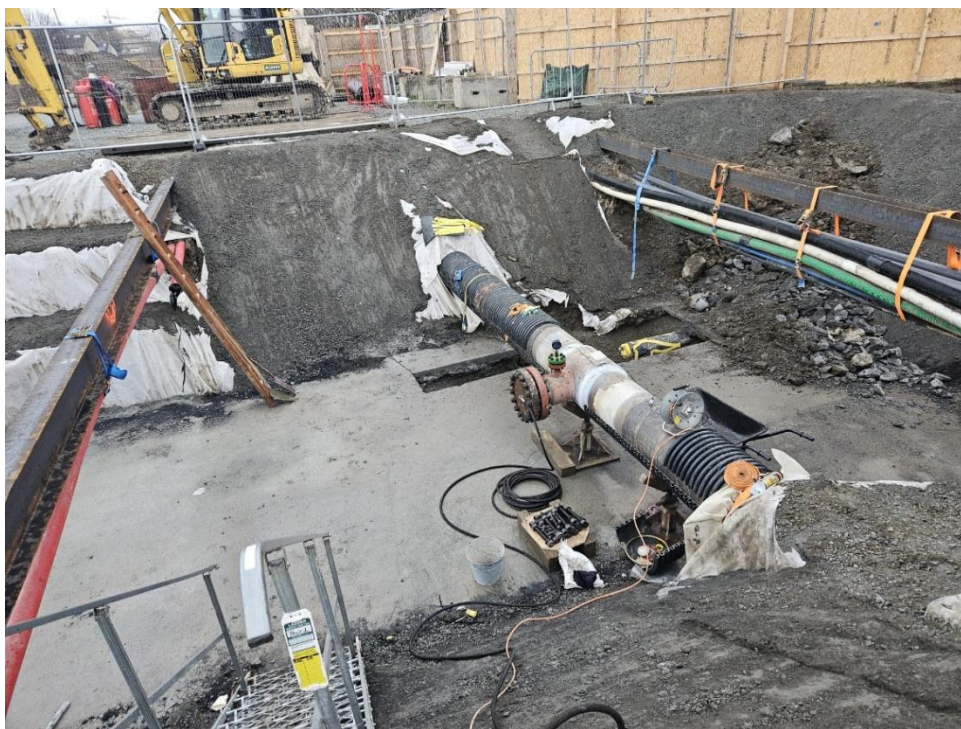
Figure 10: Hot Tap Tee Battered Excavation
