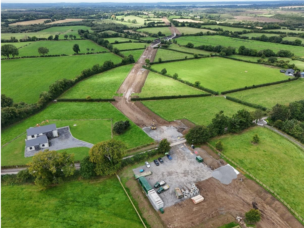
Figure 19: Typical Establishment of Laydown Area at a Road Crossing
