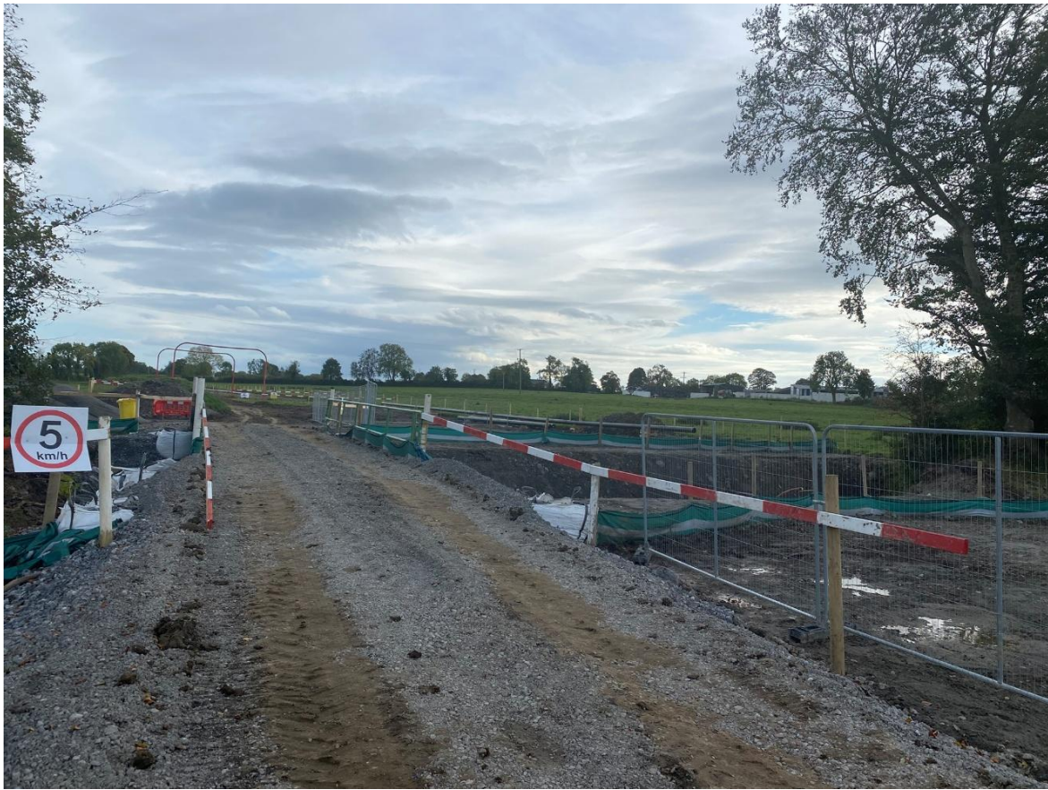
Figure 31: Bridge Crossing of Water Course.
