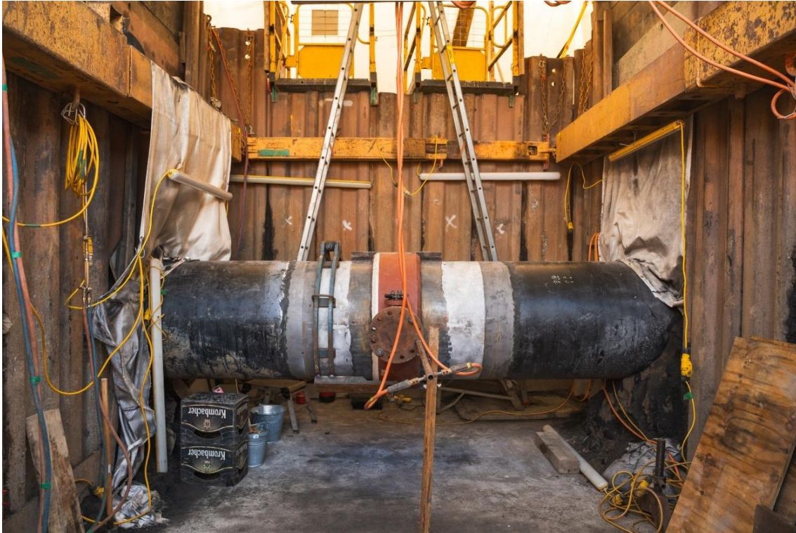
Figure 12: Hot Tap Tee Excavation Supported by Sheet Piles
