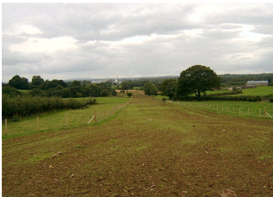
Figure 34: Image of Reinstatement of Agricultural Field Following Gas Pipeline Installation
