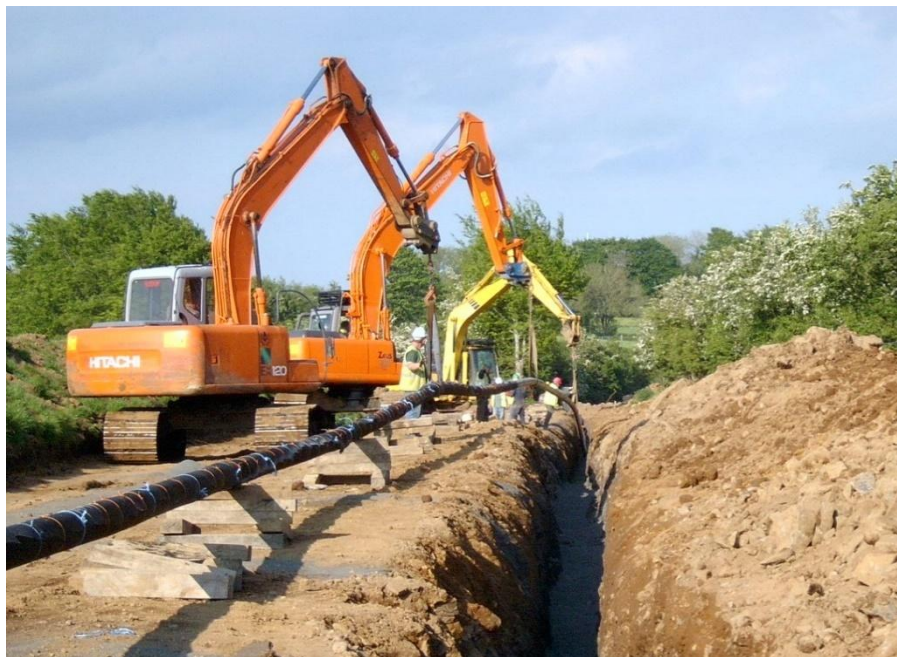
Figure 28: Image of Pipeline Being Lowered into a Trench
