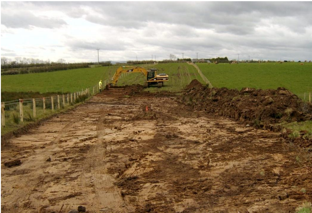
Figure 21: Image of Topsoil Removal Within Working Width
