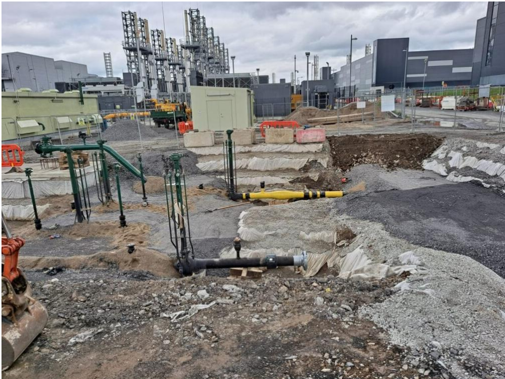
Figure 41: Typical Excavations for AGI Below Ground Pipework
