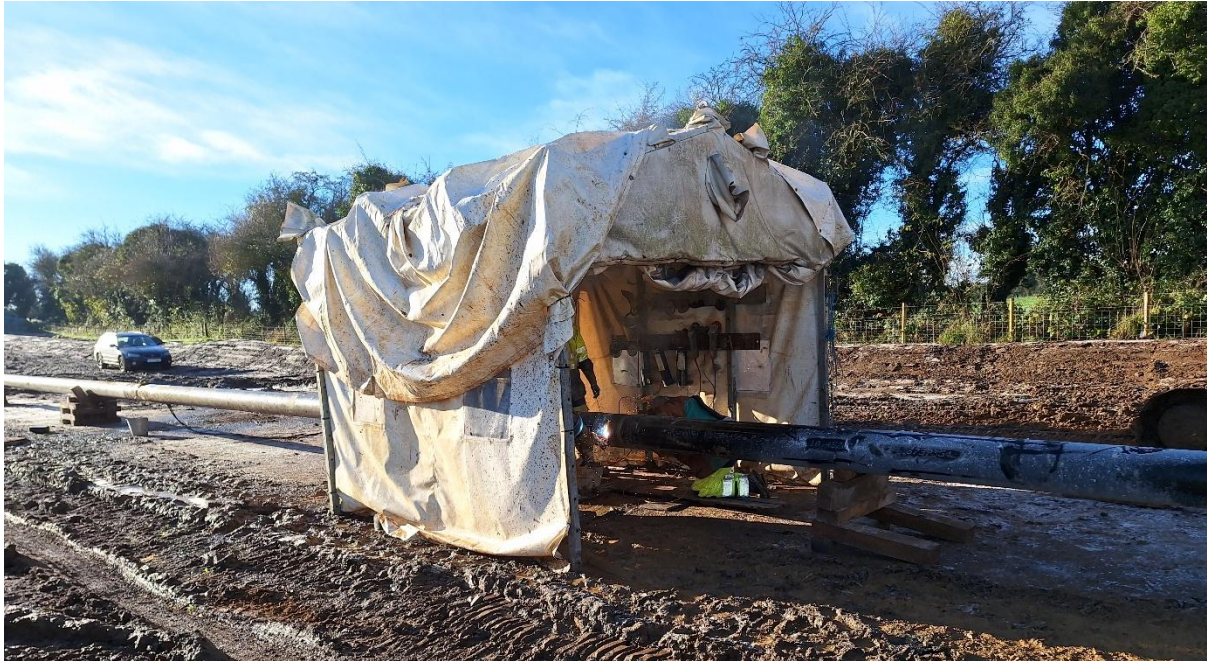
Figure 25: Welding Canopy Used for Welding Pipe Sections Together.
