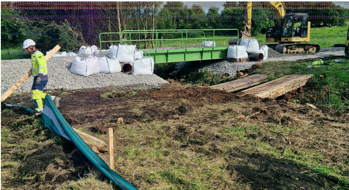
Figure 32: Temporary Bridge in Situ.
