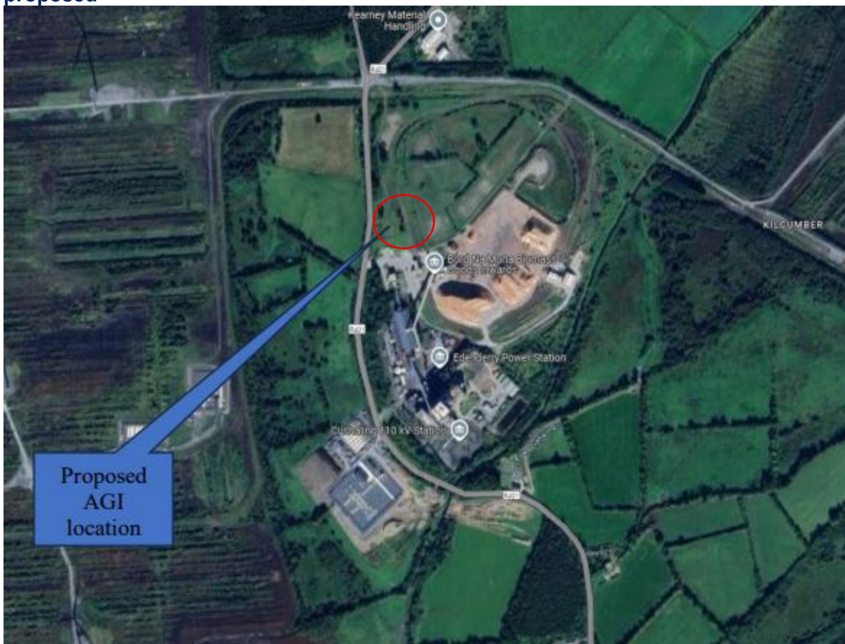
Figure 2.2: Aerial Imagery of the existing Edenderry Power Plant where the AGI is proposed
