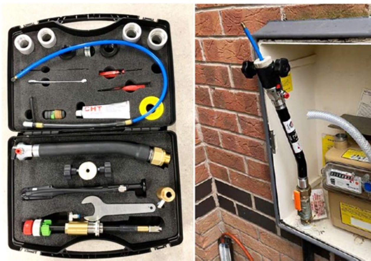
Figure 1-2: Service Connection showing the M-CEX pressure Isolation Tool.
