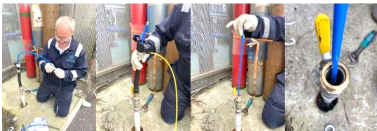
Figure 2-1: Field Trial Demonstration of Inflatable Stopper at GNI Training Centre, Dublin.
